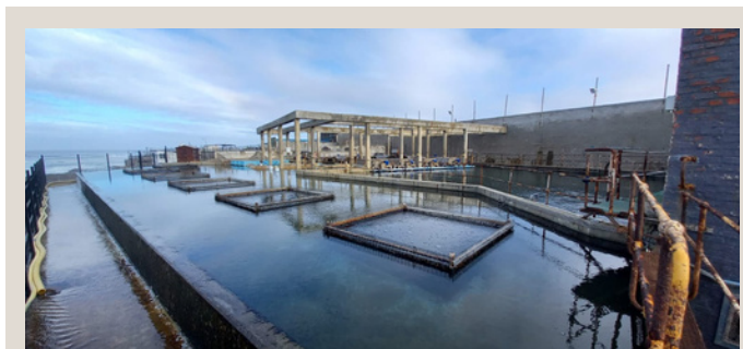
Figure 3: Primary (front) and Secondary (behind) sump at Abagold Ltd., Hermanus.
